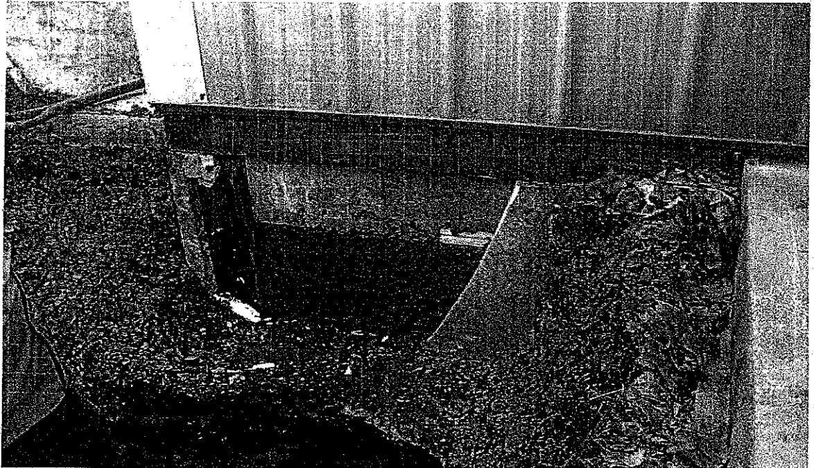
Photo 1 - West Elevation, North Corner - Foundation Test Pit
